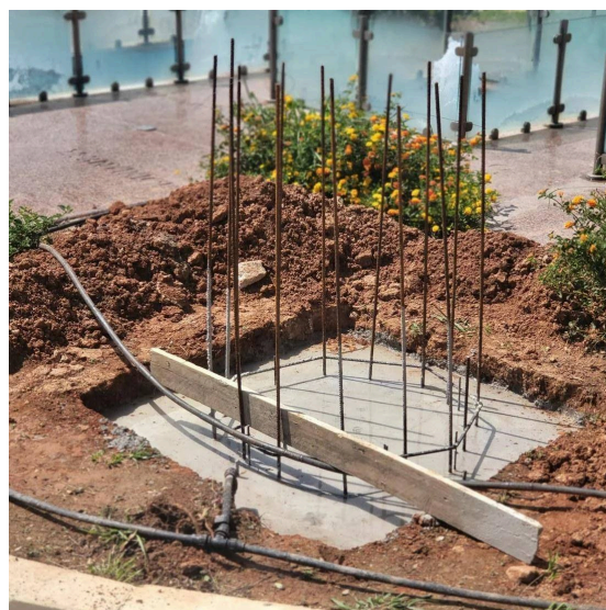
VERTICAL REINFORCEMENT ON THE FOOTING
