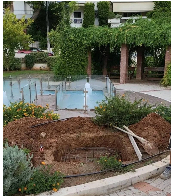
EXCAVATION AND FOOTING GRID · NEO PSYCHIKO
