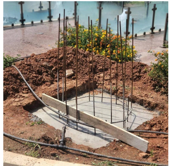
VERTICAL REINFORCEMENT ON THE FOOTING
